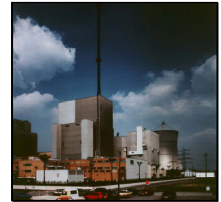
THTR: Hamm-Uentrop 300 Mwe Demonstration Reactor
